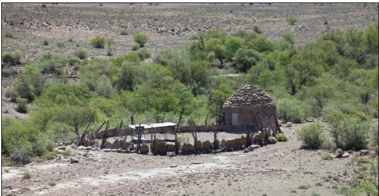
Figure 15.5: A corbelled kafhok and trapvloer, now fenced and in use as an animal pen.
