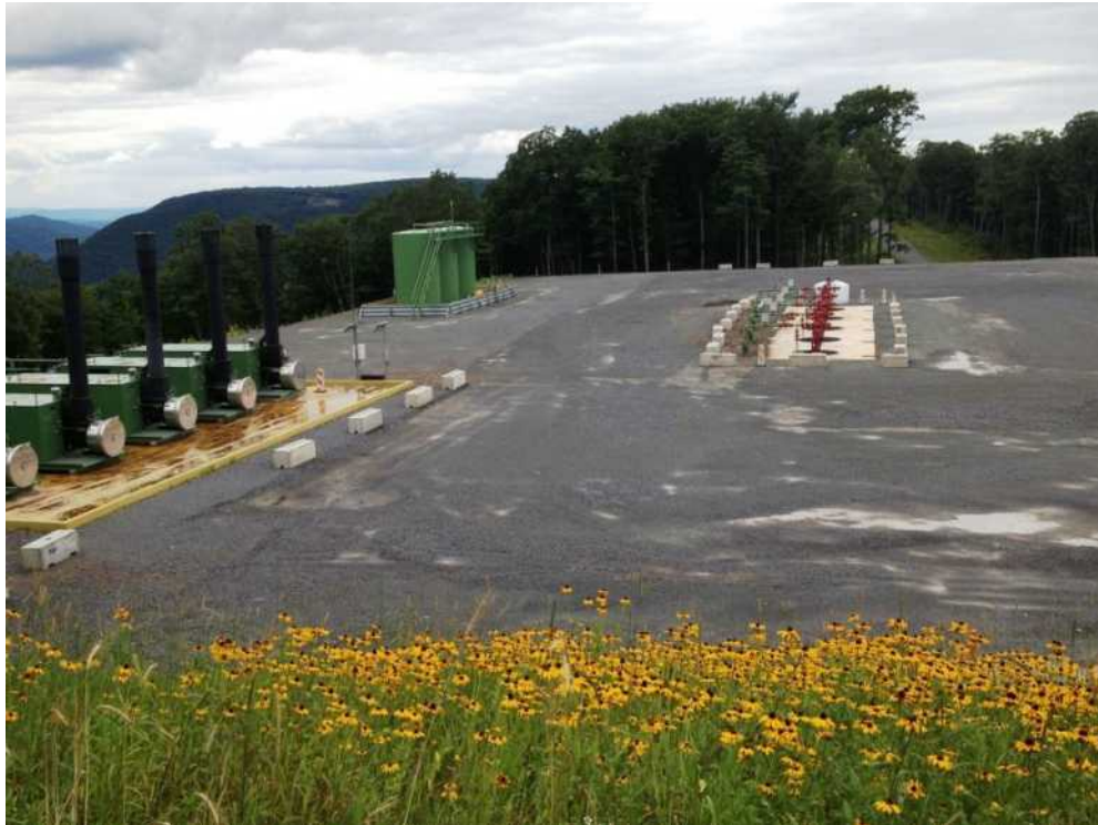
Plate 1.9: Example of a shale gas compressor station situated at a wellhead complex. Tanks used to store produced water and condensate, separated from 'wet gas', are shown located towards the top left of the plate (Source: Tom Murphy, Pennsylvania State University, USA)
