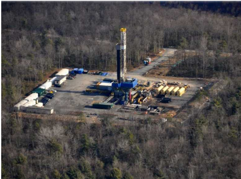
Plate 1.3: Illustration of a typical wellpad lay-out with drilling and supporting infrastructure in place (Source: Tom Murphy, Pennsylvania State University, USA).
