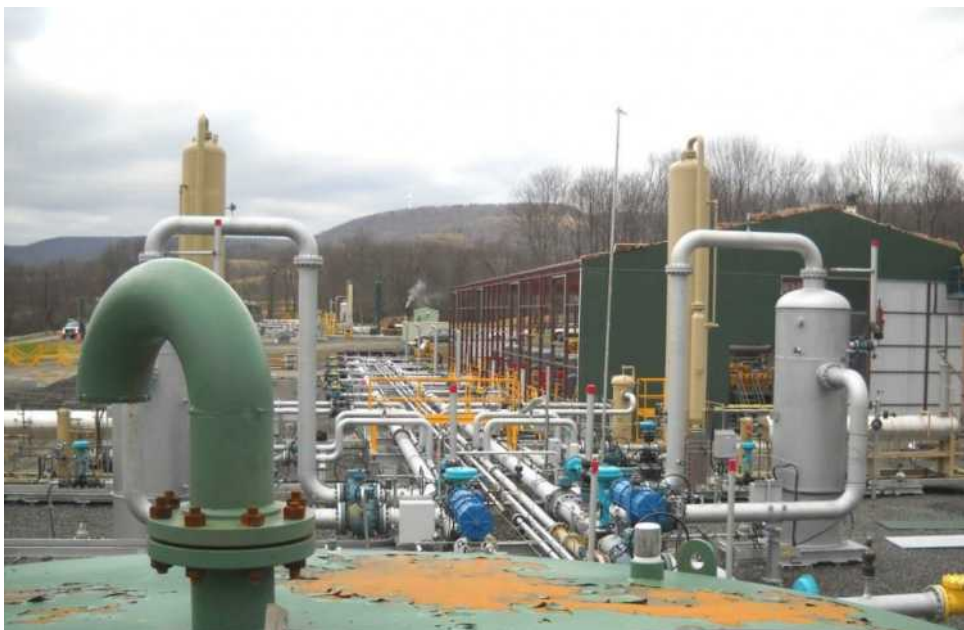
Plate 1.10: Example of a centralised gas compressor station. Compressed gas would be exported from this facility, via pipeline, to a downstream facility such as a CCGT power station (Source: Tom Murphy, Pennsylvania State University, USA)
