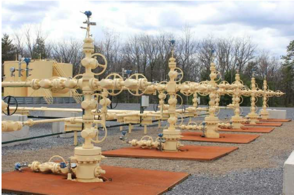
Plate 1.8: Cluster of producing wellheads (Source: Tom Murphy, Pennsylvania State University, USA)
