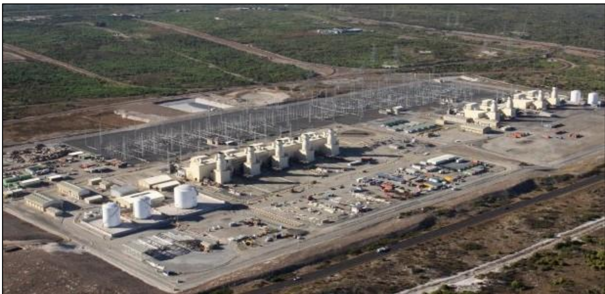
20 21 Figure 2.7: Existing Open Cycle Gas Turbines (OCGTs) at Atlantis, South Africa (9 x 148 MW, 1 327 MW 22 Ankerlig power station) currently running on diesel (Eskom Holdings SOC Ltd n.d.). Similar plants will be part 23 of new OCGT capacity planned for in the IRP 2010 but will run on natural gas. 24
